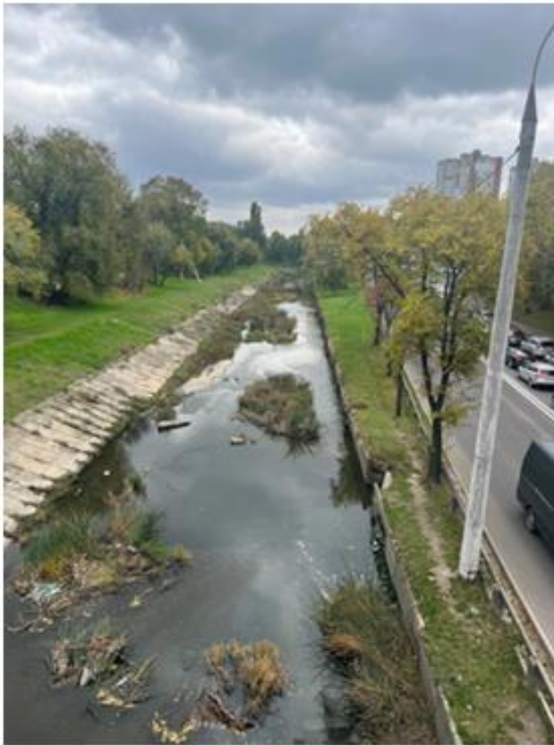
Perspective of the Bîc River and Albișoara Street from the Renasterii Nationale Bridge
